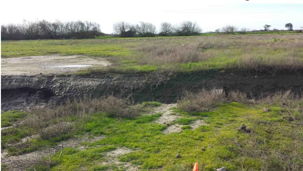
New South Channel Cross section 3 -SC3. View is looking south.
