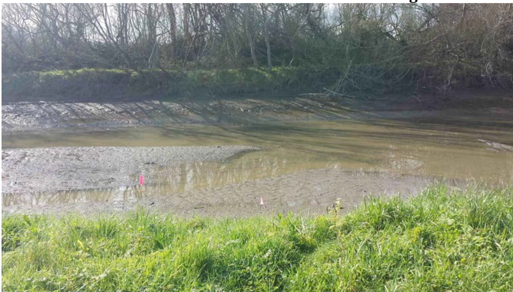
Salt River Channel Cross section 3 –SR3. View is looking south.
