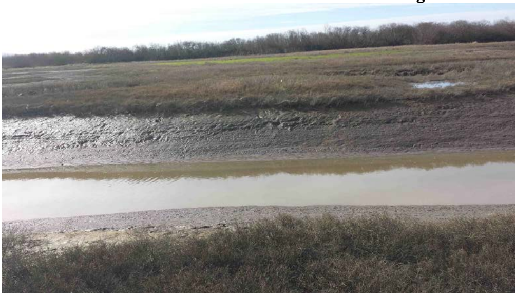
New South Channel Cross section 2 -SC2. View is looking south.
